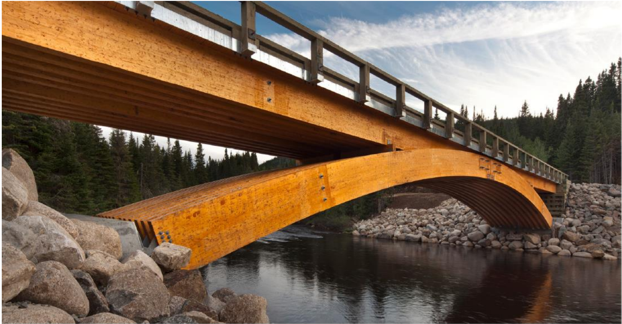
FIGURE 2: MASS TIMBER BRIDGE REDUCES THE USE OF CONCRETE AND STEEL.
