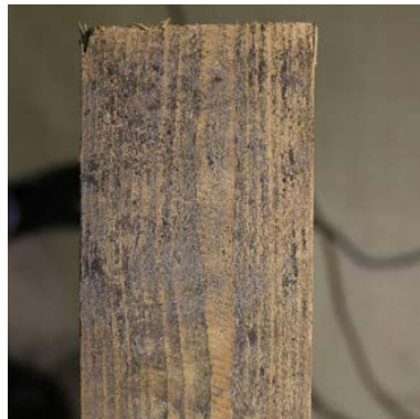
Figure 5. CW Formwork wood – original image
