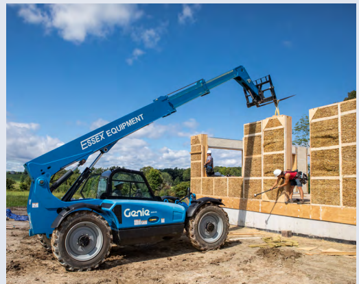
Installation of prefabricated straw panels. Courtesy of New Frameworks.
