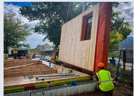
Timber Age Modular Building System (TAMBS) panels made from cross-laminated timber. Courtesy of Timber Age Systems
