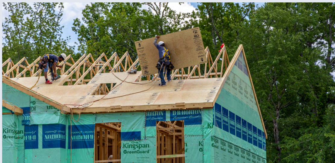
Installation of Plantd panels. Courtesy of Plantd, https://www.newswire.com/news/plantd-signs-multi-year-contract-with-d-r-horton-for-10-million-carbon-22444348
