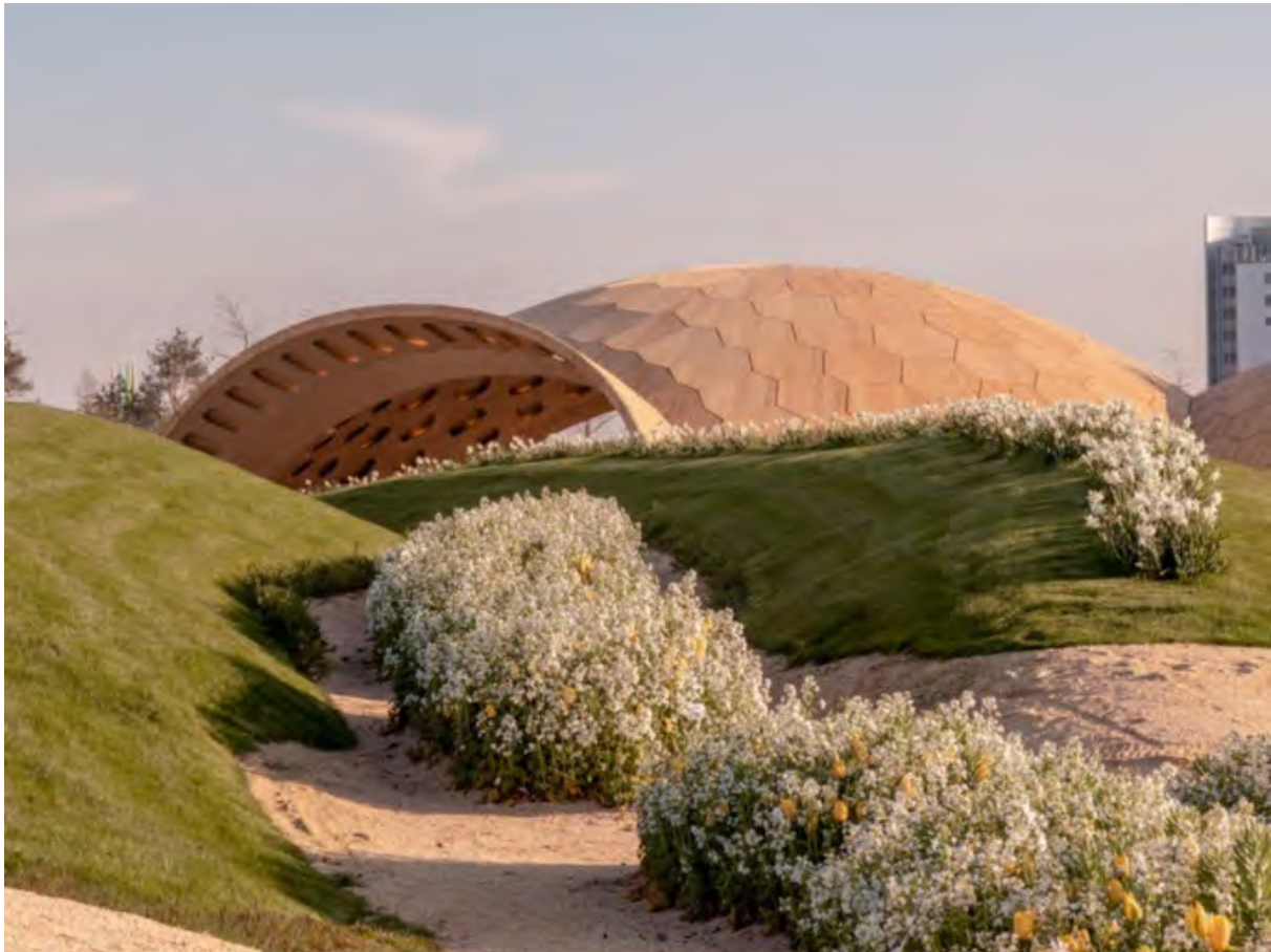
Figura 58. Vista exterior Wood Pavilion 2019
