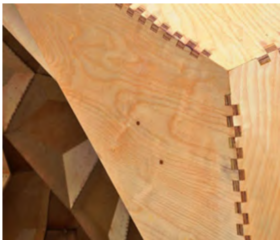
Figura 33. Detalle juntas Research Pavilion 2011
